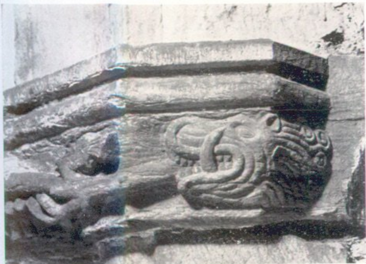
West crossing arch. 1513 × 1588.
