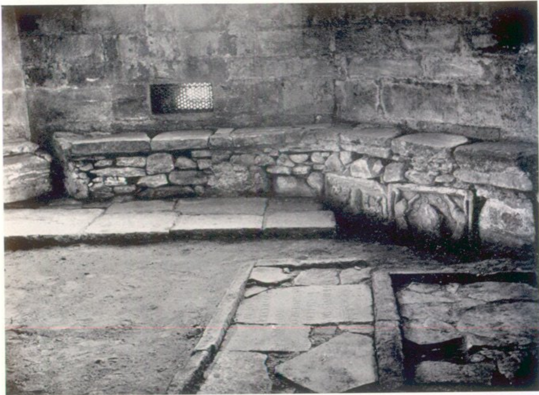
The chevet: lower floor and "benching".
