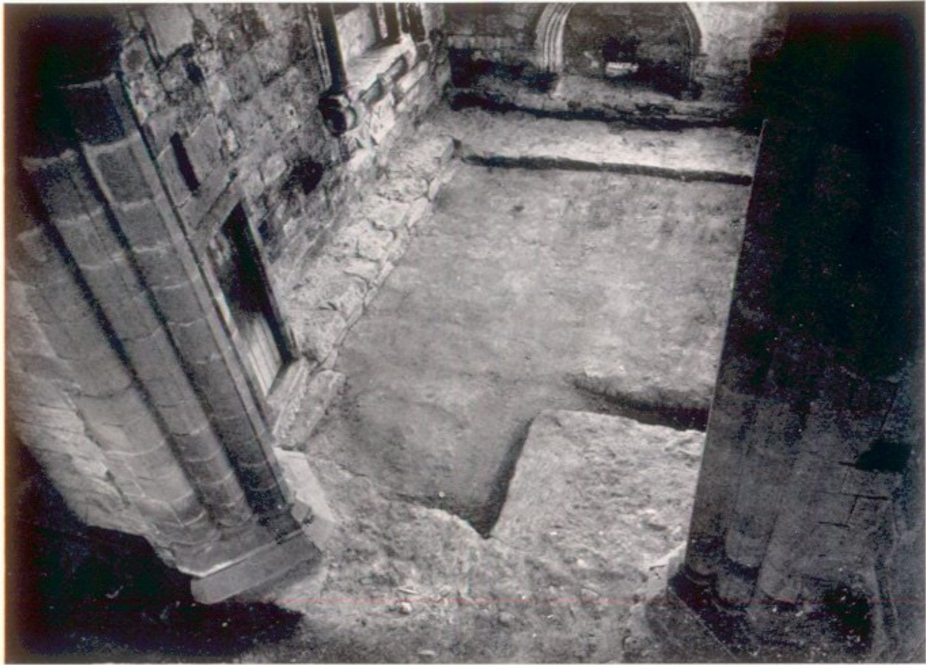
The south transept from the crossing tower showing older foundations. (See plan.)
